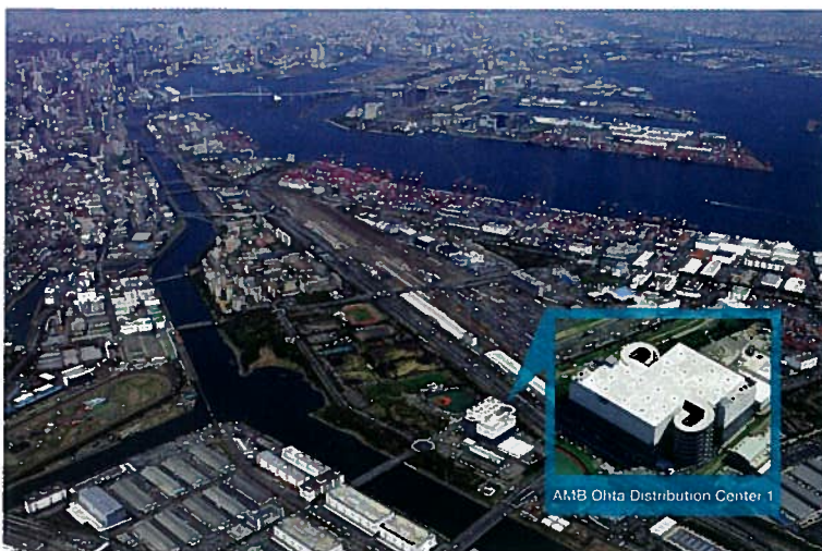
The seven-story AMB Ohta Distribution Center at the Port of Tokyo has a floor/area ratio in excess of 398 percent.
