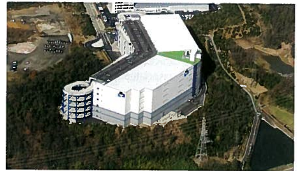
Multistory distribution centers, prevalent in the industrial hubs of Tokyo, Osaka, Singapore, and Hong Kong, would be a workable solution to lessening the carbon footprint in the United States. In Nagoya, Japan, AMB Property Corporation was able to preserve 60 percent of the trees on a 705,000-square-foot (65,496-sq-m) parcel by building a six-story distribution center.
